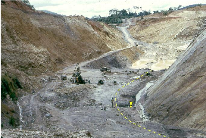
**Figure 3 | View of the open pit of Oklo during exploration of the reactors (1973).** The top-left limit of the C1 uranium-rich layer is indicated by the yellow dashed line. An arrow points to the top of Reactor 2 to the right of the person standing in the area cleared for scientific studies.
