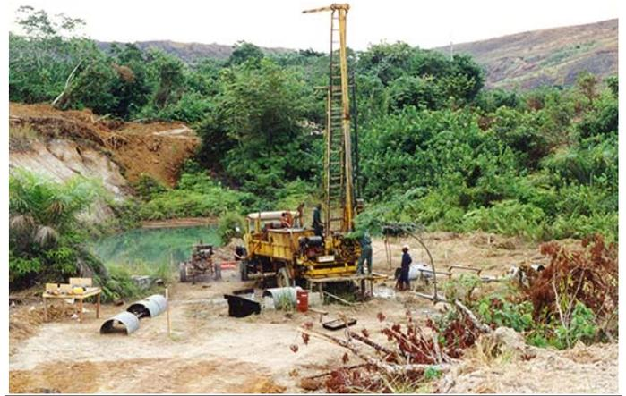
**Figure 7 | View of the Bangombé reaction zone during the drilling exploration (1996).** It is the last natural nuclear reactor known. There are no pictures of this reactor since it was preserved. These boreholes produced the evidence for the existence of this reactor.
